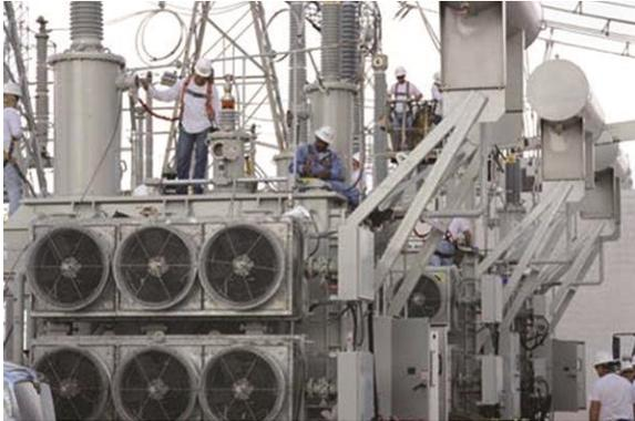
**4. A resilient prototype.** Three single-phase extra-high-voltage transformer prototypes developed with backing from the Department of Homeland Security under the Recovery Transformer (RecX) project were field tested from 2012 to 2013 at a CenterPoint substation near Houston, where they continue to operate. The field test demonstrated RecX's rapid deployment speed. It was transported, installed, and energized in less than six days. *Source: DHS/Paul Wedig*
